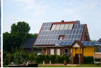
solar system storage
